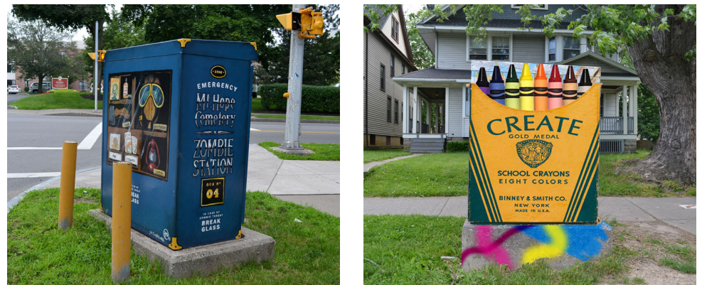
Figure 9.8 - Painted Electric Box as a Creative Way and Cost-Effective Way to Make Infrastructure Elements Unique and Add to the Sense of Place
