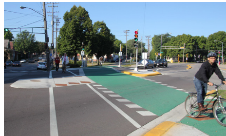
Figure 5.11 - Clearly Defined/Visible Trail Crossing at Roadway
