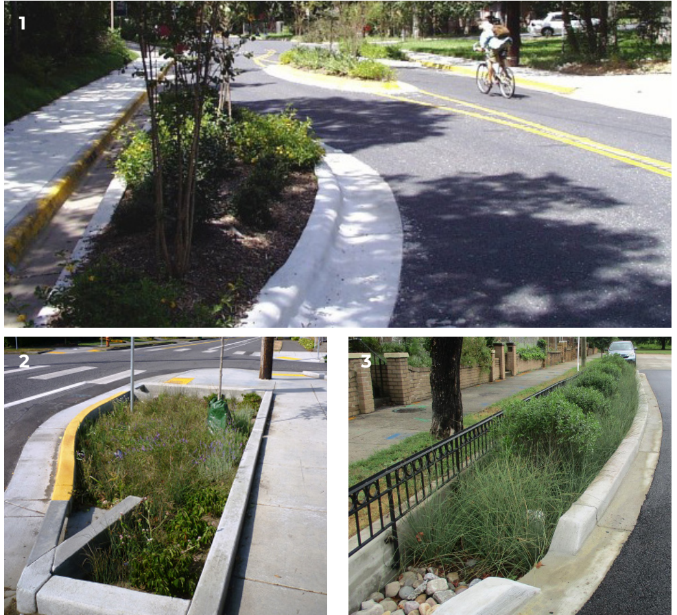
Figure 6.25 - Examples of Traffic Calming Elements such as Chicanes (1), Landscaped Bump-Outs Incorporating Green Stormwater Infrastructure (2 and 3)
