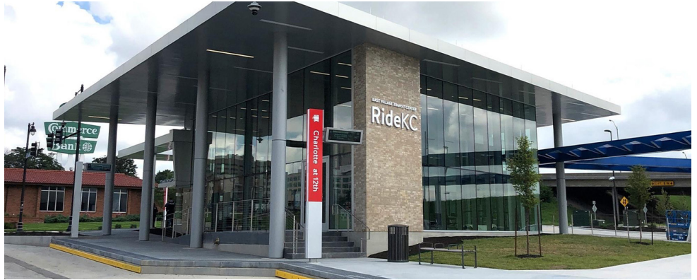
Figure 6.32 - RideKC East Village Transit Center - Charlotte Street/12th Street
