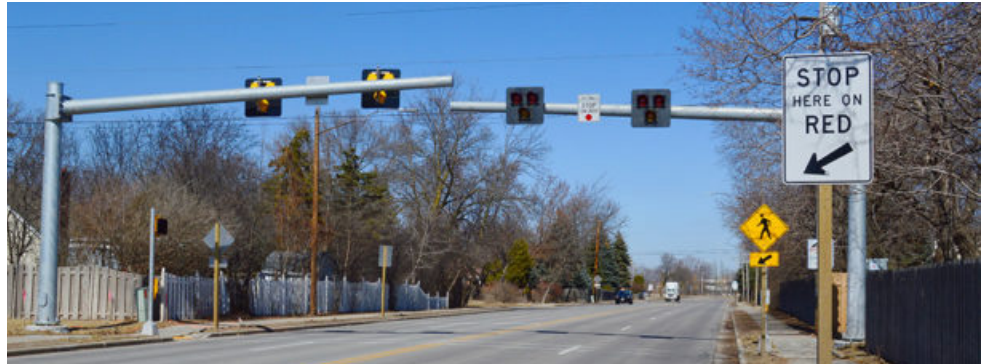
Figure 6.5 - HAWK Beacon for Mid-Block Pedestrian Crossings
