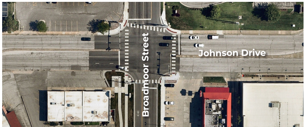
Figure 7.28 - Pedestrian Improvements Made to Johnson Drive/Broadmoor Identified as "Average Conditions" by the Steering Committee
