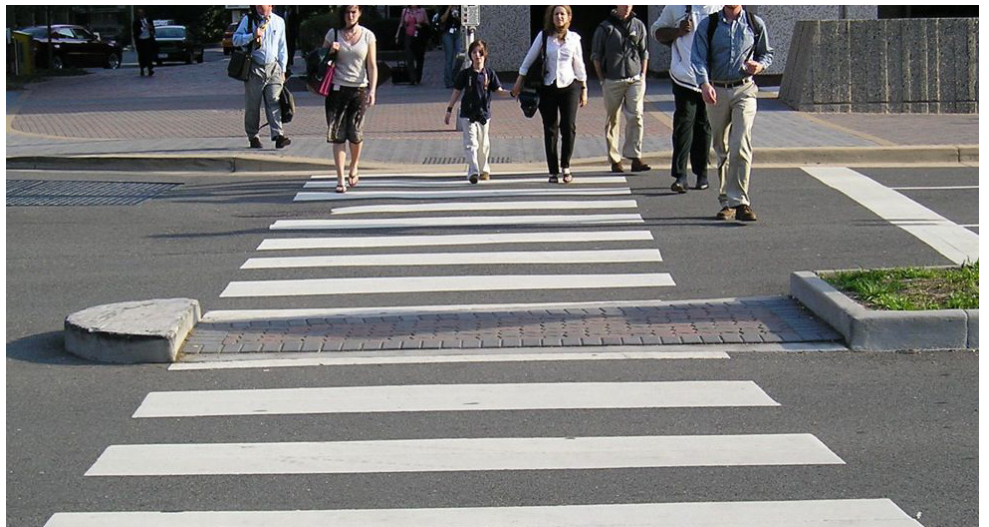
Figure 7.18 - Example of a Well-Marked Crosswalk
