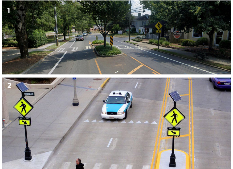
Figure 6.28 - Examples of Pedestrian Refuge Island (1) and Rapid Rectangular Flashing Beacons (2)
