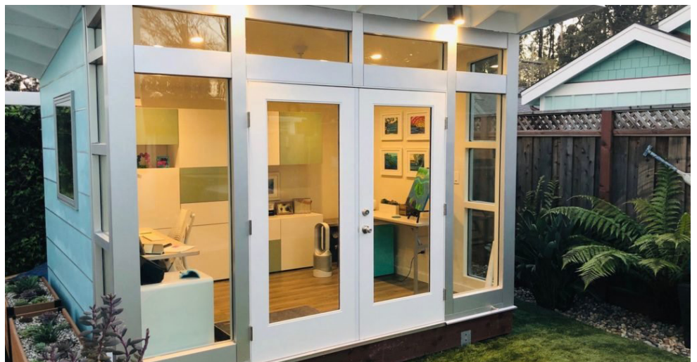
Figure 7.16 - Accessory Office Structure
