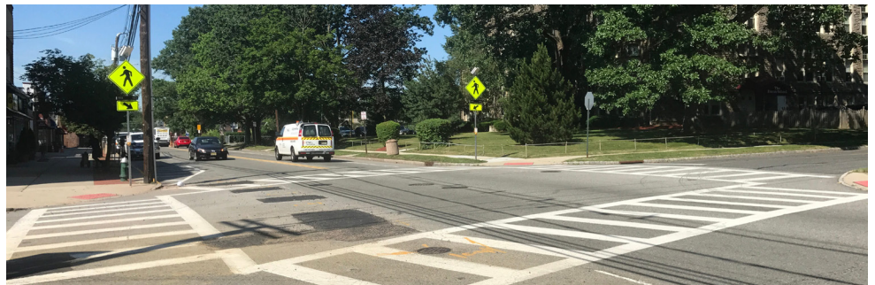
Figure 6.6 - Well-Marked Pedestrian Crosswalks
