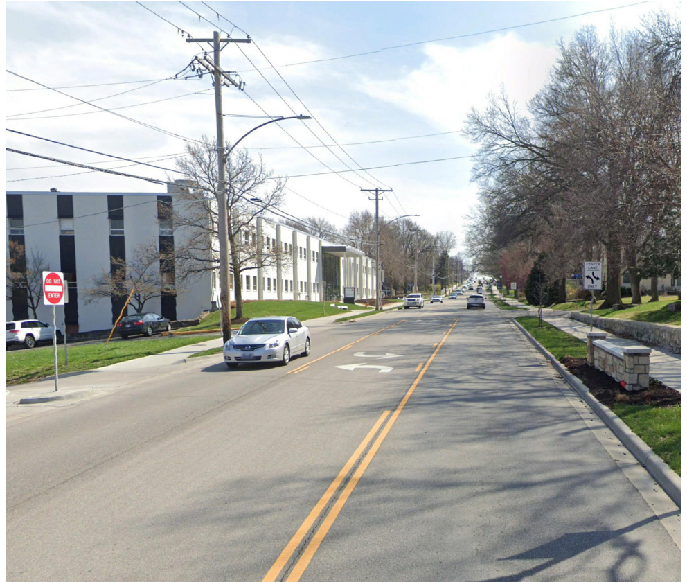
Figure 6.26 - Roadway Corridor in Johnson County that Recently Experienced a Road Diet and went from 4-Lanes to 3-Lanes
