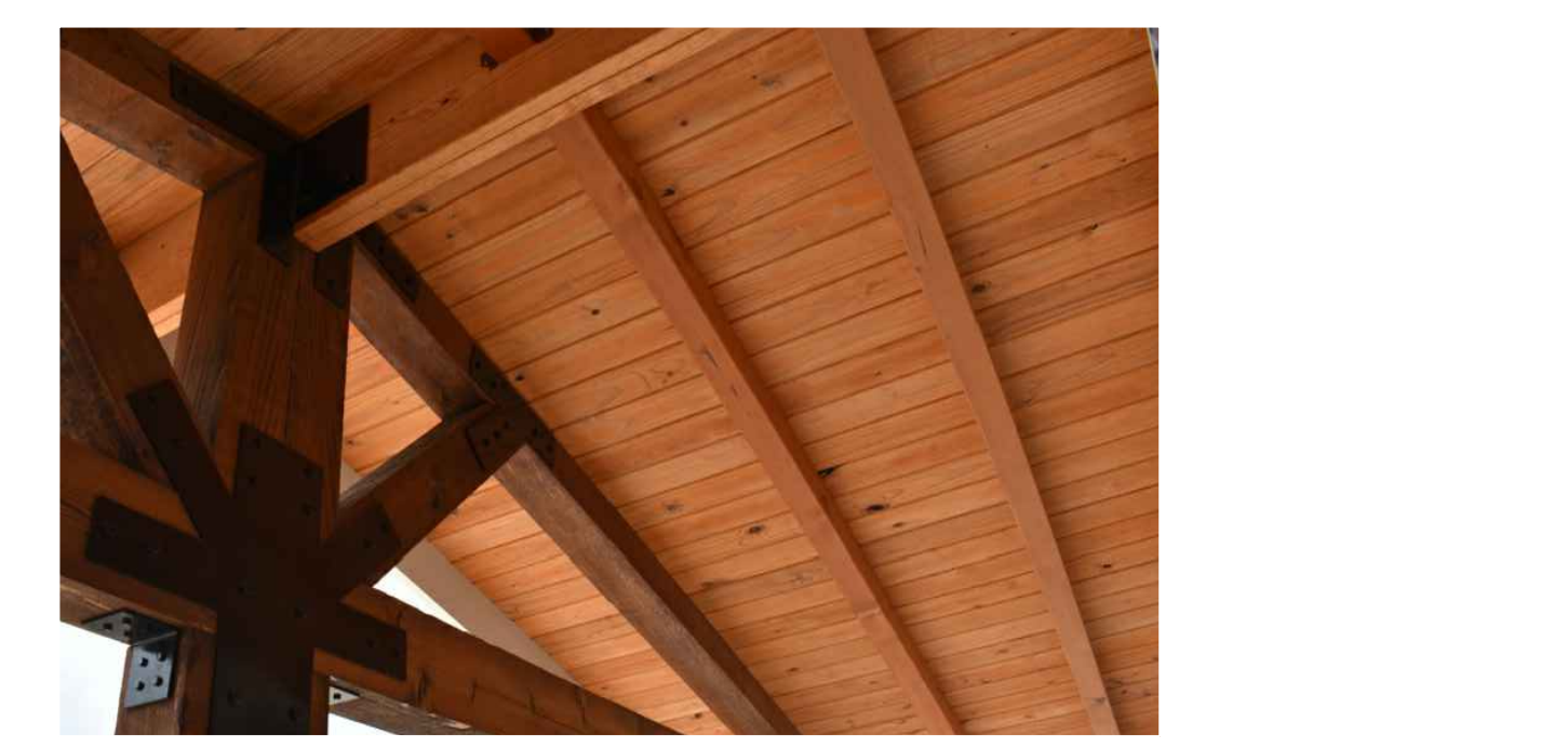
WOOD MATERIAL MATERIAL: DOUGLAS FIR COLOR: REDWOOD LOCATION: RESTROOM CEILING
