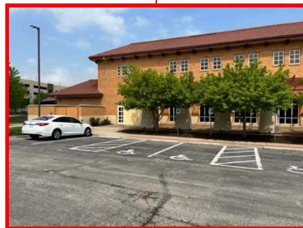
ALTERNATIVE LOCATION 2: LOCATE CHARGING STATIONS ON WEST SIDE OF BUILDING NEAR EXISTING ACCESSIBLE SPACES AND CLOSE TO UTILITY TRANSFORMER.
