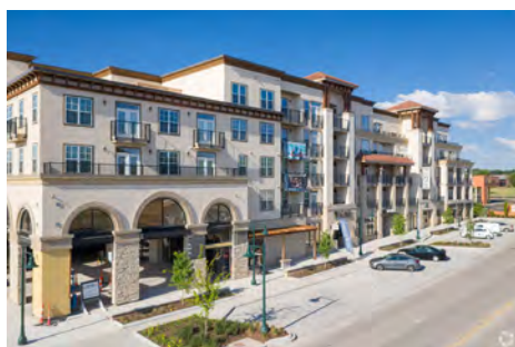
Figure 7.11 - 'The Locale' Mixed-Use Development on Johnson Drive
