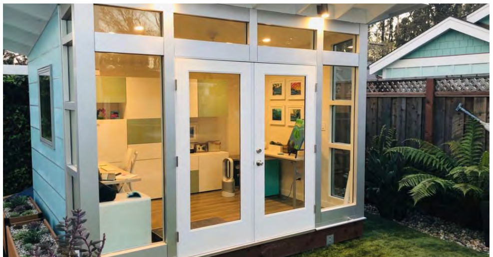
Figure 7.16 - Accessory Office Structure
