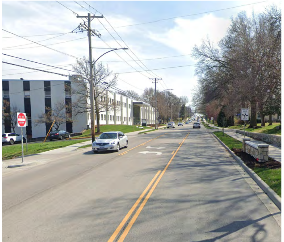
Figure 6.24 - Roadway Corridor in Johnson County that Recently Experienced a Road Diet and went from 4-Lanes to 3-Lanes
