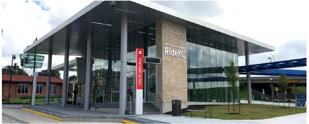
Figure 6.30 - RideKC East Village Transit Center - Charlotte Street/12th Street
