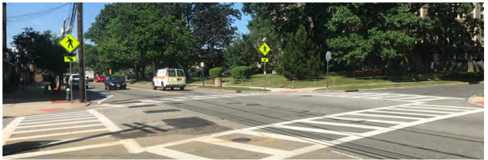
Figure 6.6 - Well-Marked Pedestrian Crosswalks
