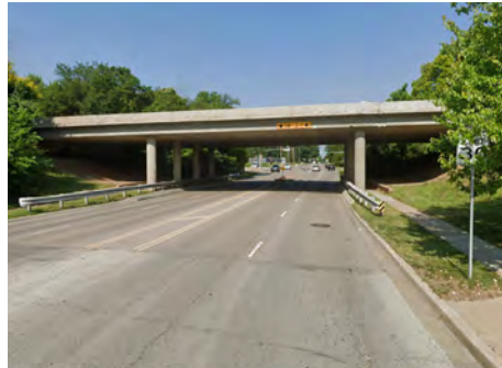
Figure 6.32 - Existing Conditions at Metcalf Avenue as Viewed From Johnson Drive
