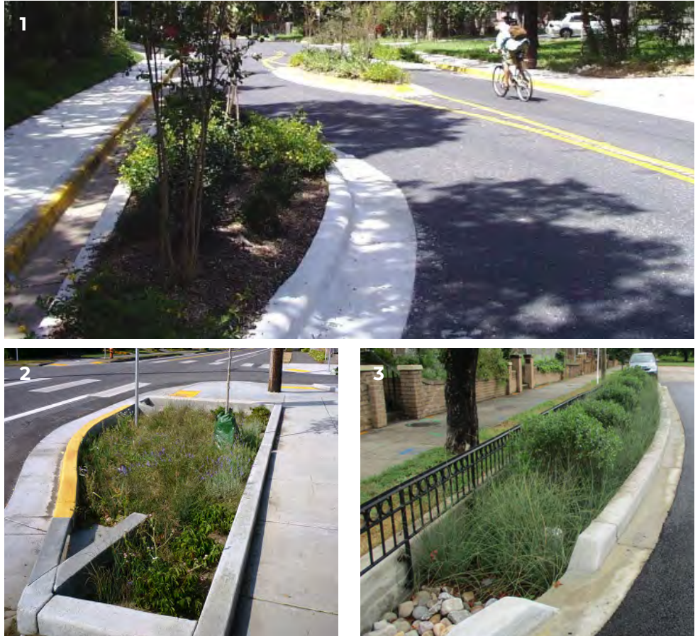
Figure 6.23 - Examples of Traffic Calming Elements such as Chicanes (1), Landscaped Bump-Outs Incorporating Green Stormwater Infrastructure (2 and 3)
