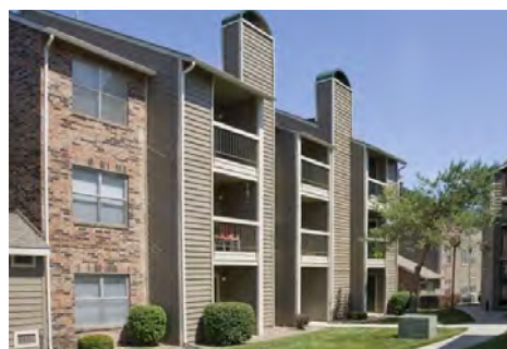
Figure 8.32 - Apartments in Mission
