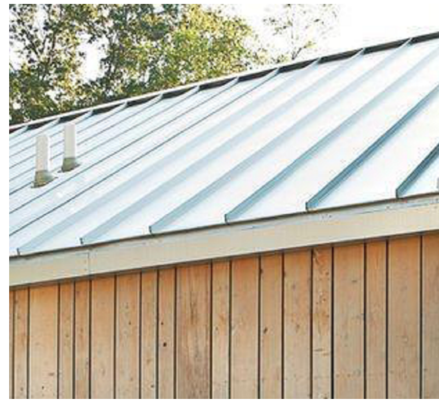
STANDING SEAM METAL ROOF
