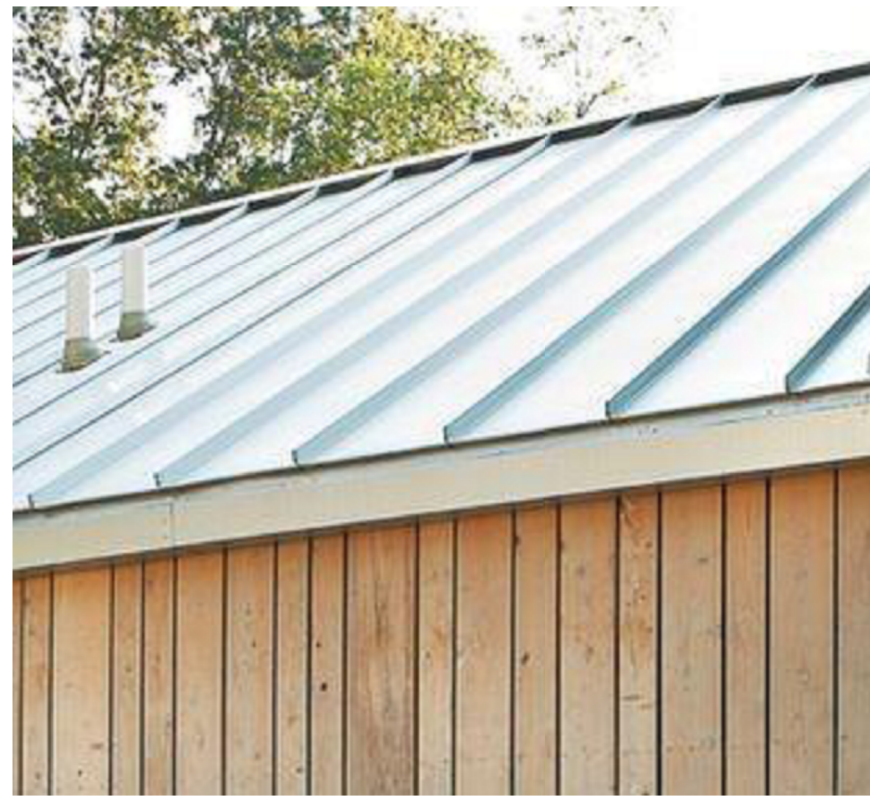
STANDING SEAM METAL ROOF
