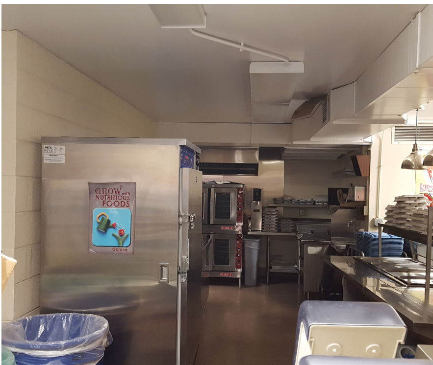
Low head clearance in Kitchen
