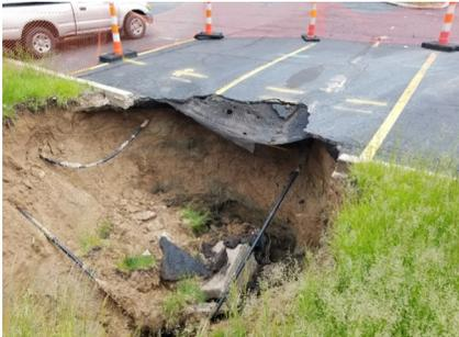
The heavy rains this spring continue to point out the challenges of an aging stormwater infrastructure system throughout the City. BHC Rhodes has been working with staff to improve our asset inventory related to the stormwater conveyance system, taking existing inventory and condition rating data and combining it into maps and databases.
