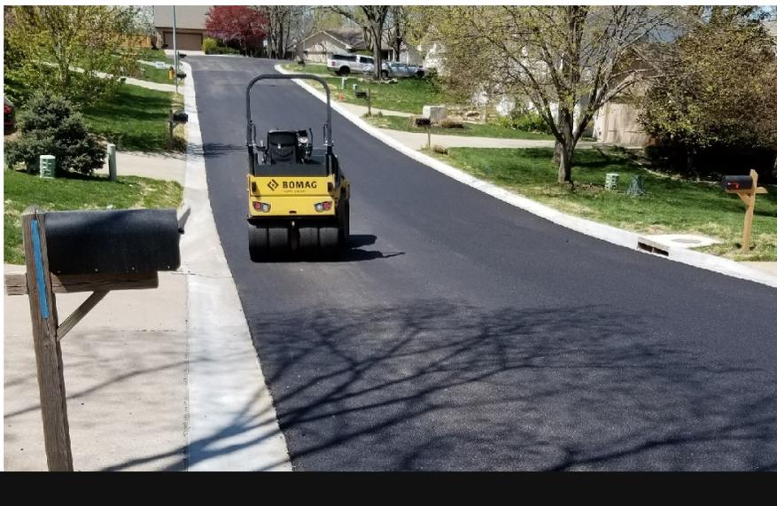
*Little Joe's Asphalt completed the mill and overlay of 52nd Terrace (west of Lamar Ave) earlier this week. This project was a carry over from last fall as the contractor was not able to get the project completed before the weather turned too cold.*
